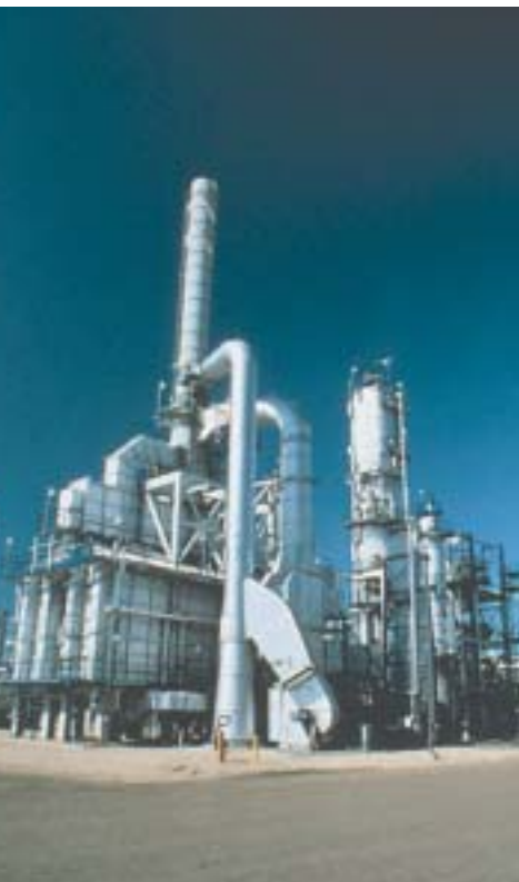
Figure 16-2 An Oil Refinery The crude oil is processed in large refineries.
